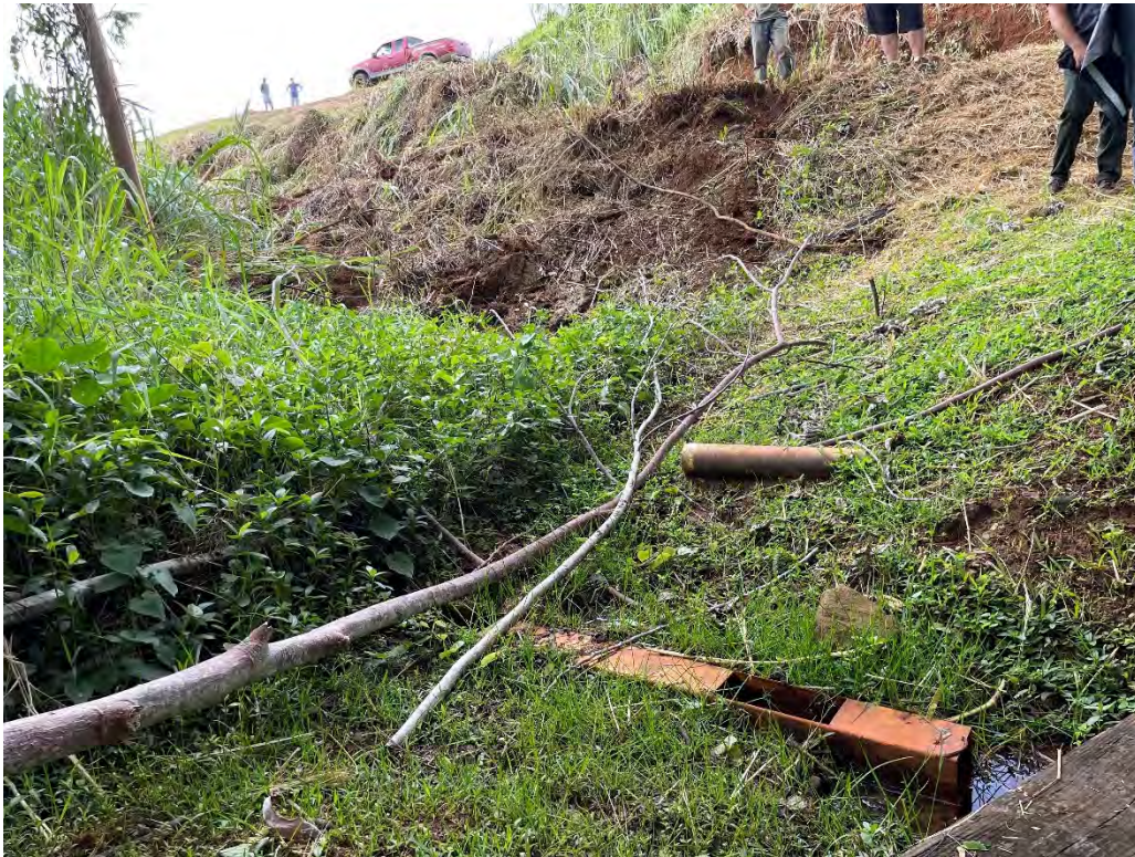
Photo B-24: Seepage Flume (S-1) at Downstream Toe of Right Embankment Segment (looking upstream and slightly right at left end of right embankment segment).
