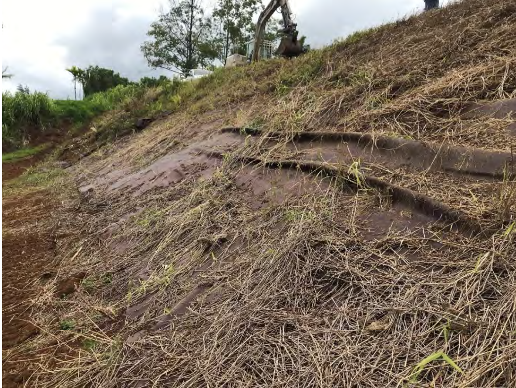
Photo 2-6: Erosion Mat along Downstream Embankment Slope. Looking towards Right Abutment
