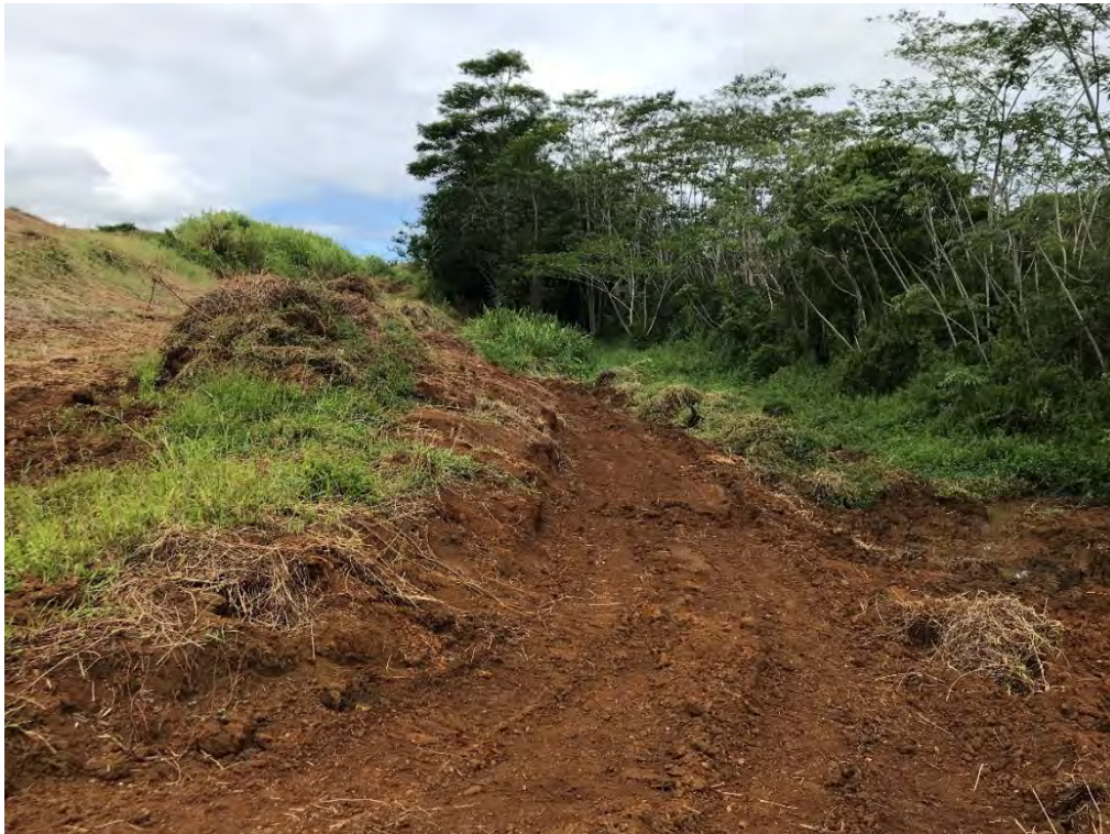
Photo B-26: Downstream Embankment Toe (cleared for inspection, looking left toward left end of right embankment segment)
