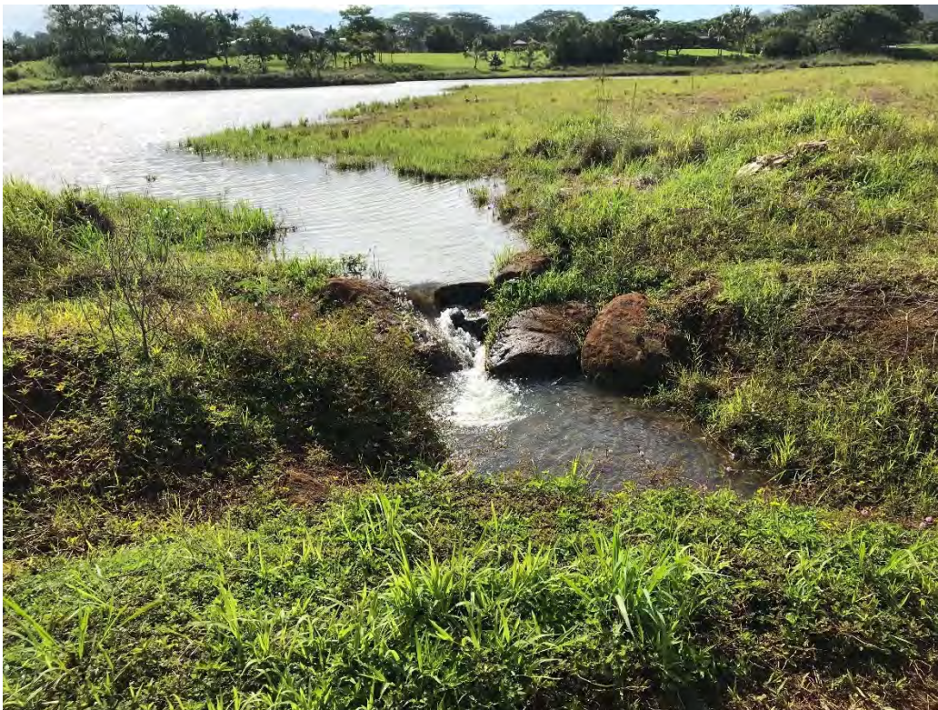
Photo B-32: Approach to Mid-level Outlet Near Left Abutment (Standing Above Two 24-inch Diameter HDPE Culverts)
