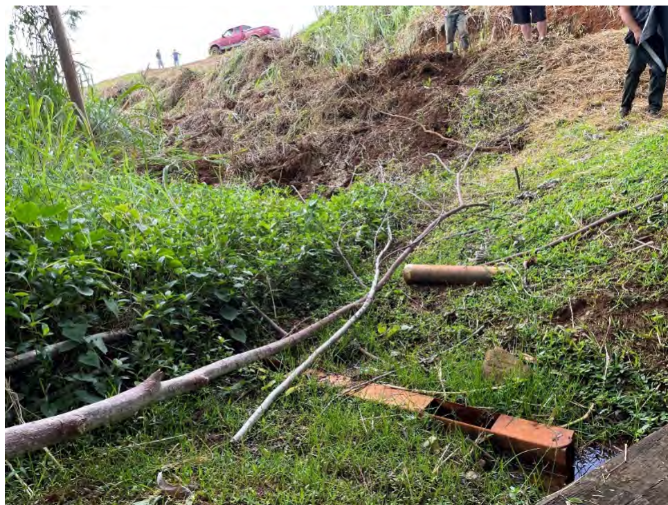
Photo 2-16: Flume to Monitor Seepage at Downstream Toe of Right Embankment Segment
