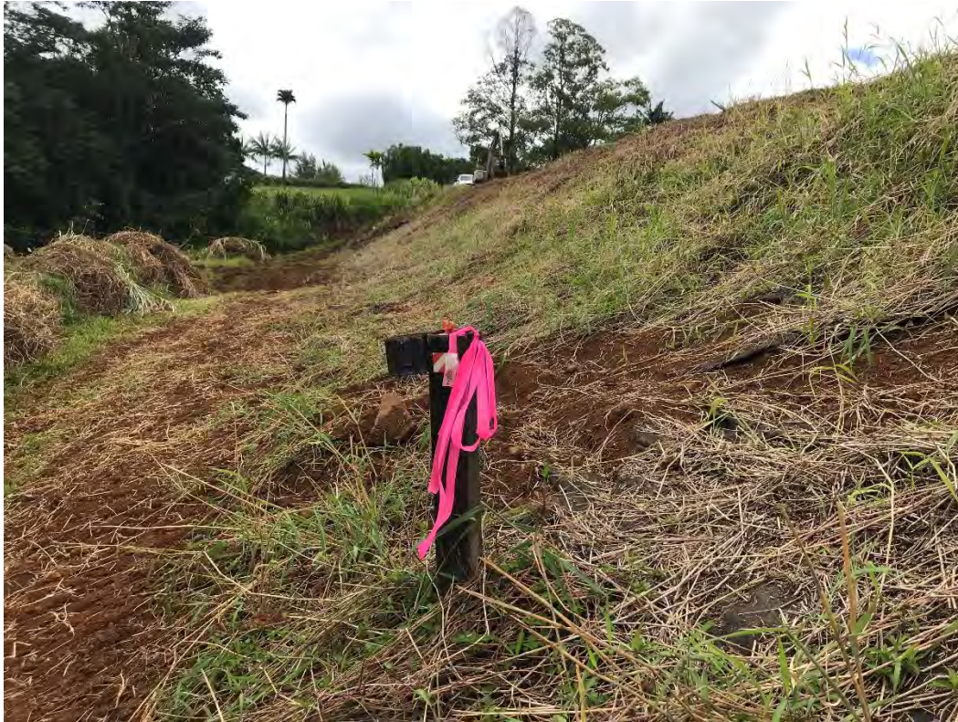
Photo B-19: Piezometer PZ-1 at Downstream Embankment Slope, Right Embankment Segment (looking right)
