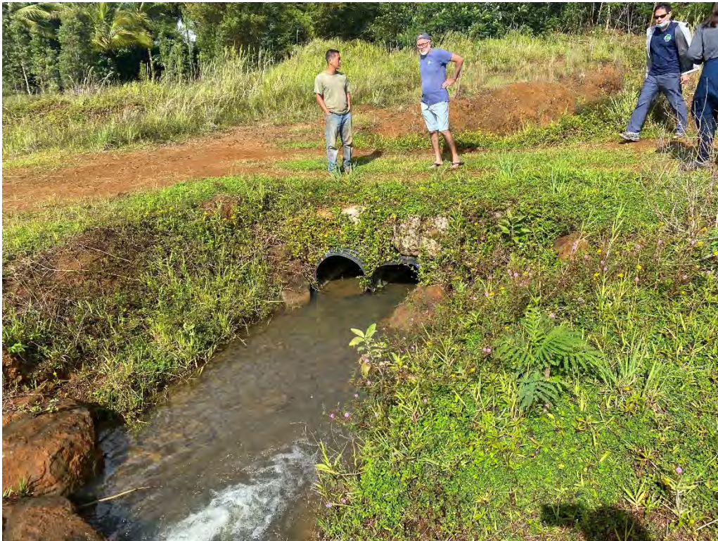
Photo B-30: Mid-level Outlet Structure (Two 24-inch Diameter HDPE Culverts)
