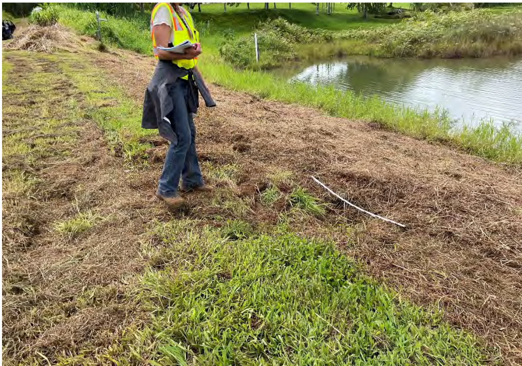
Photo B-12: Depression in Dam Crest on Right Embankment Segment (reportedly from brush removal)
