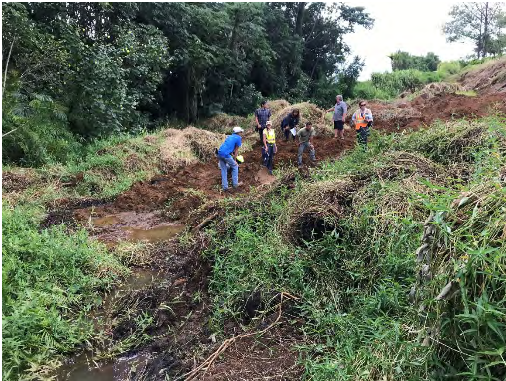
Photo B-28: Seepage Collection Ditch along Downstream Toe of Right Embankment Segment (looking right)
