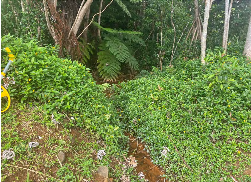
Photo B-25: Area of Seepage along Downstream Toe of Right Embankment Segment (looking downstream from Seepage Flume)
