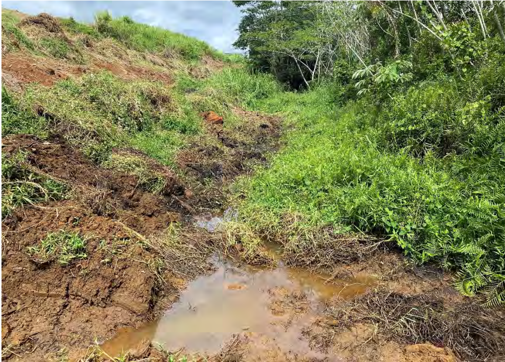
Photo B-27: Seepage Collection Ditch along Downstream Toe of Right Embankment Segment (looking toward left end of right embankment segment)
