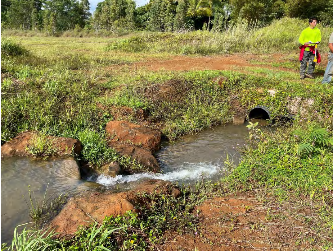
Photo B-33: Rock Control Section to Mid-level Outlet Near Left Abutment
