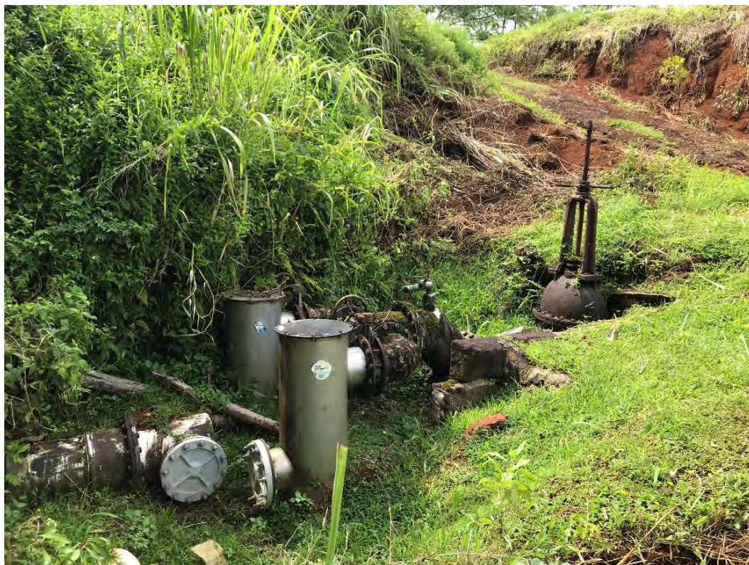
Photo 2-10: Low Level Outlet Works Valve at Downstream Embankment Toe (Outlet #1)
